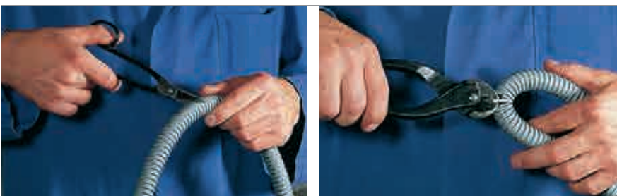
Couper le gainage synthétique Cut through the plastic sheathing
